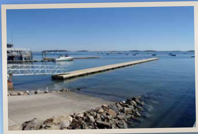
To left: the addition of riprap to the boat ramp and an aluminum gangway in Quincy.
